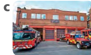
at a fire station
